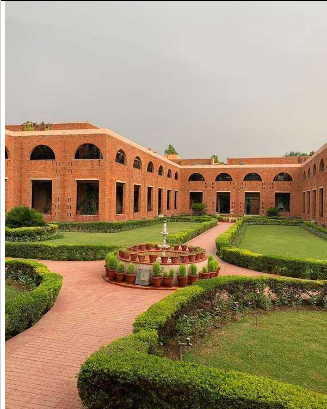
Gyan Grih - Academic Complex, Library building, MDI Gurgaon
