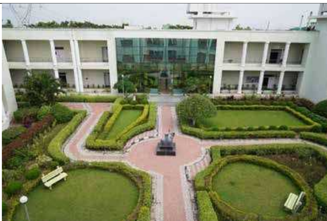
Ariel View of Building
